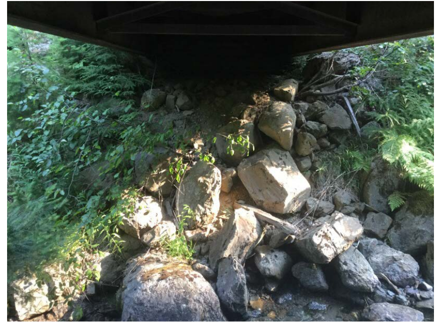
Right Bank Abutment when facing downstream
