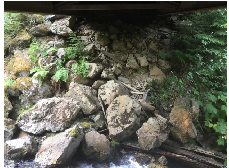
Left Bank Abutment when facing downstream
